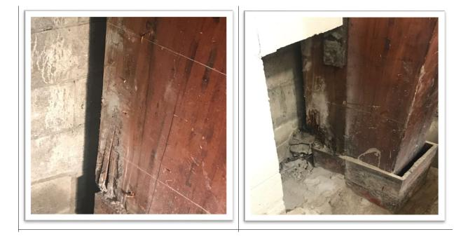
1. <u>Structural Wood Beam Delamination and Deterioration</u>
