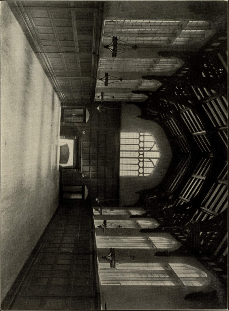
EASTERLY END OF HALL, SHOWING ENTRANCE AT LEFT AND MONUMENTAL FIREPLACE
